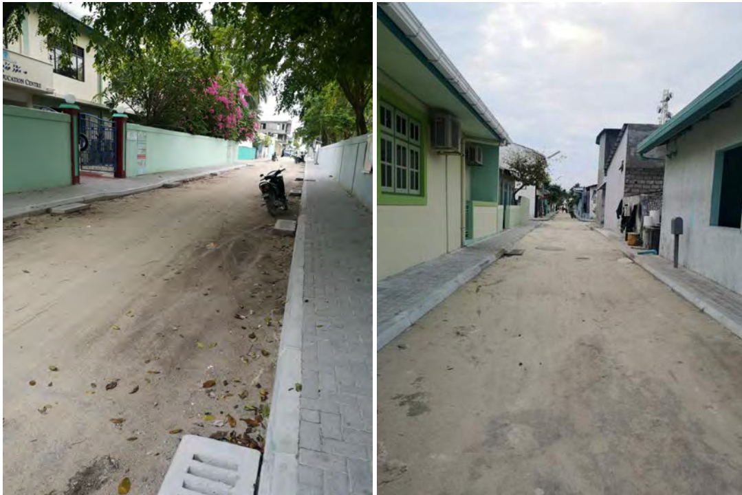
Figure 18 Road conditions in B. Eydhafushi
