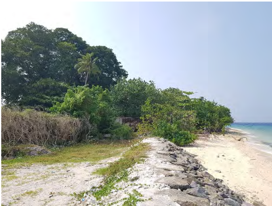
Figure 6 End point of revetment
