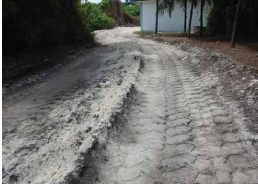
Figure 22: Impact on roads from heavy vehicle transport in an island in Maldives
