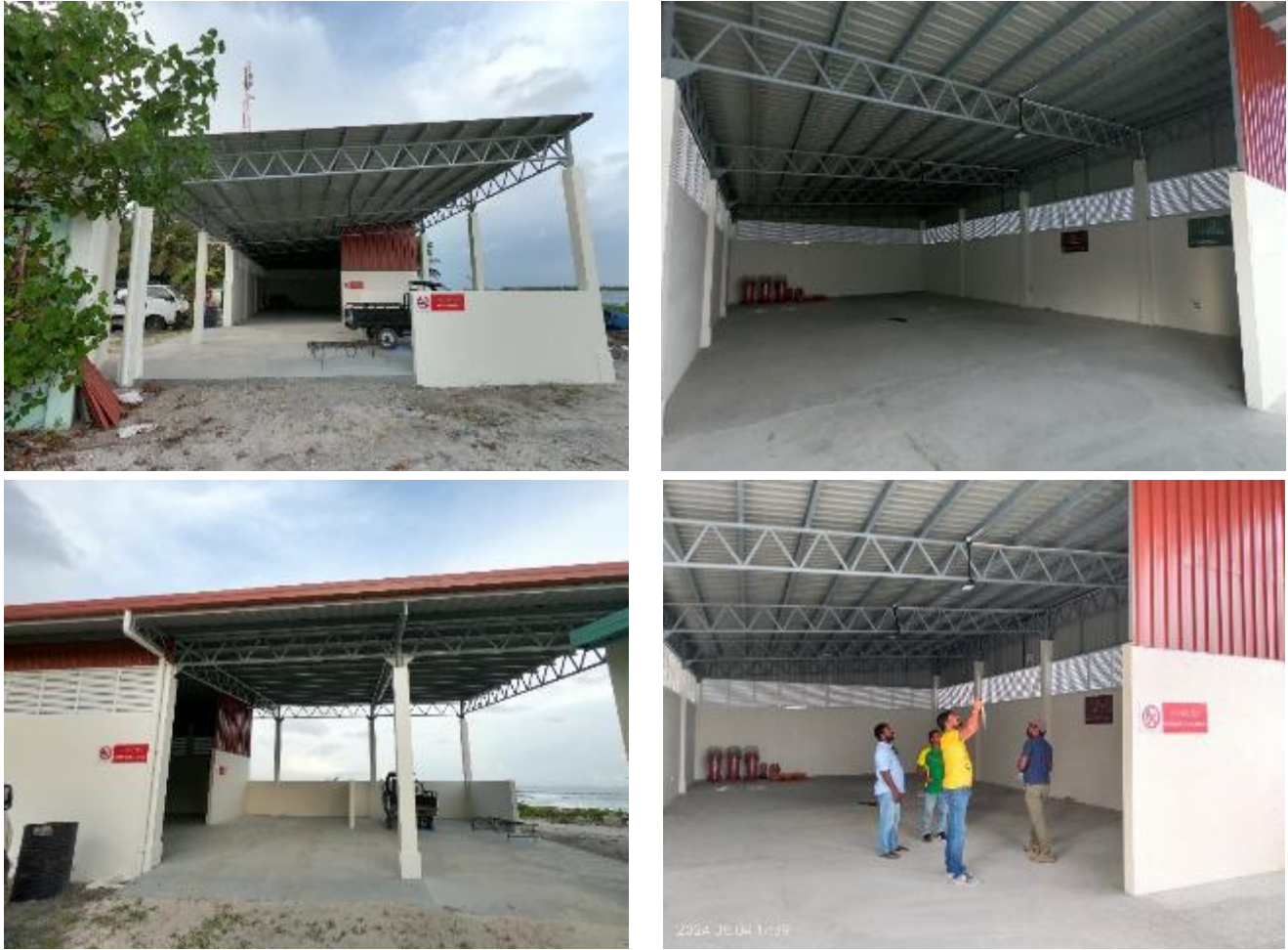
Figure 3. Photographs of upgraded IWRMC in L. Maamendhoo.
