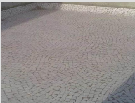
Cool Roof through China Mosaic
