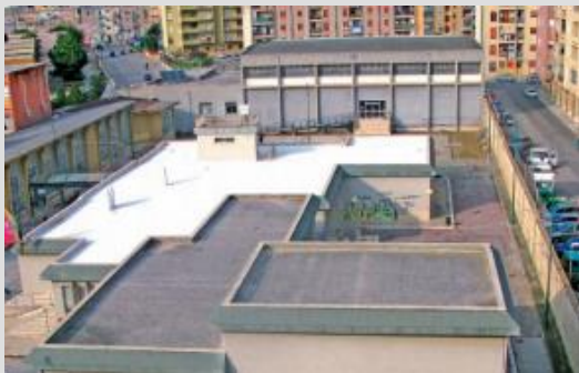
Cool Roof through white Coating
