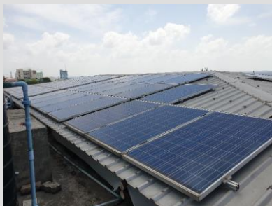
Use of solar photo voltaic roof top system for electricity generation
