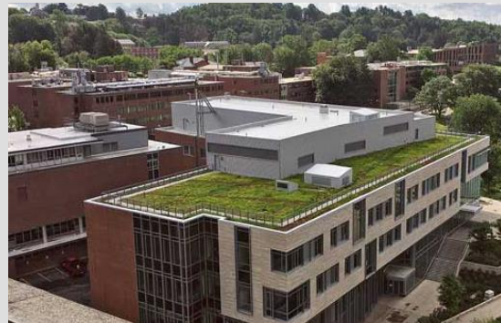
Cool Roof using Landscaping
