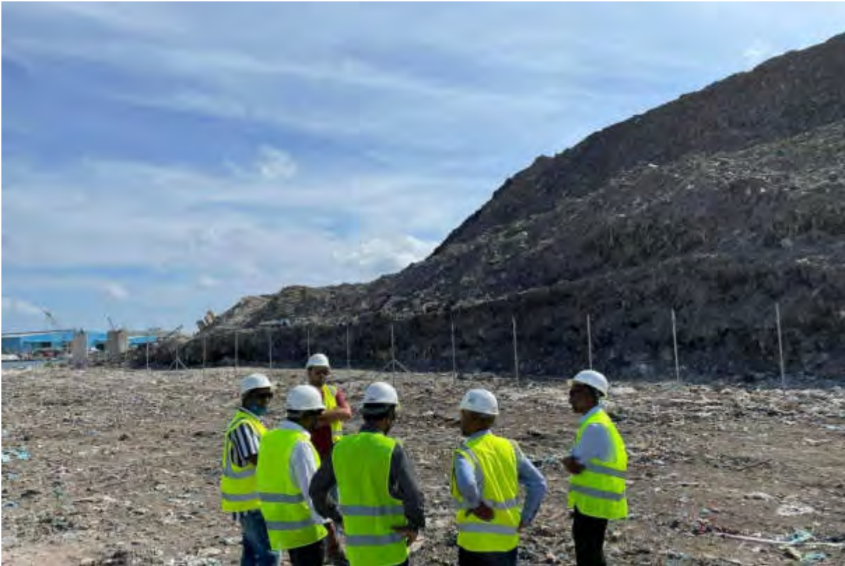
MoE, FIT and URB representatives visited the site and held the meeting regarding to landfill activities by WAMCO.
