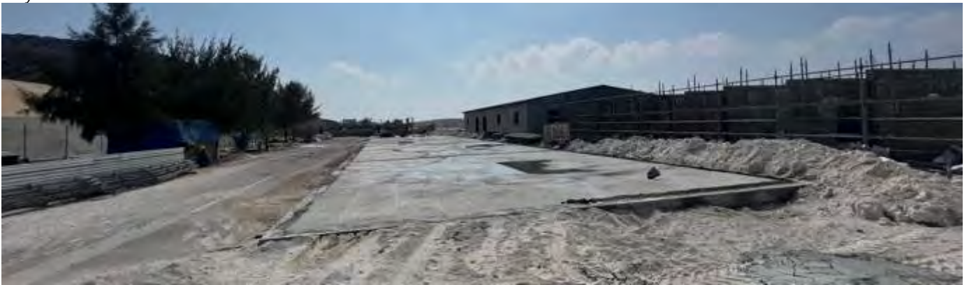
Photo 12 by Naahee 18/02/23 09:40hrs. Construction of temporary facilities, workers accommodation building ongoing.
