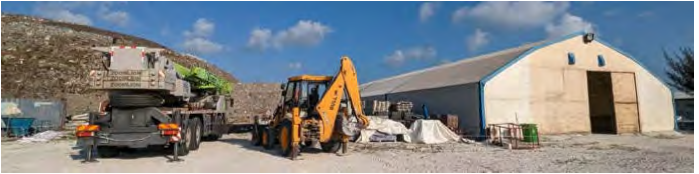
Photo 35 by Naif 27/02/23 16:56hrs Storage area and some heavy machinery on site.
