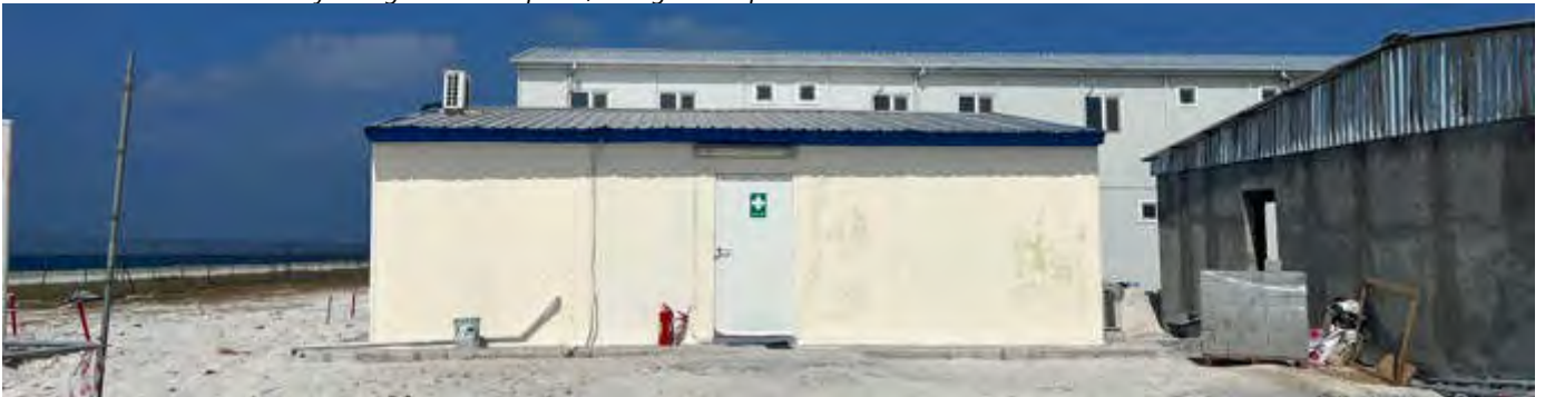
Photo 21 by Naahee 18/02/23 09:51hrs. Site first aid room/clinic and doctors and nurse on site at all times when work is carried out.
