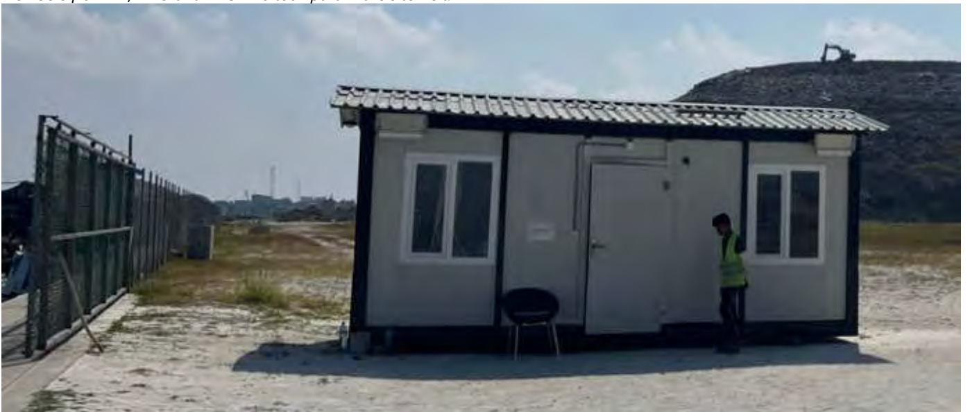
Photo 29 by Naahee 18/02/23 10:08hrs Manned security guard post, at the entrance gate on the seaside quay wall area, this is where the speed boat offloads all workers on and visitors onto site.
