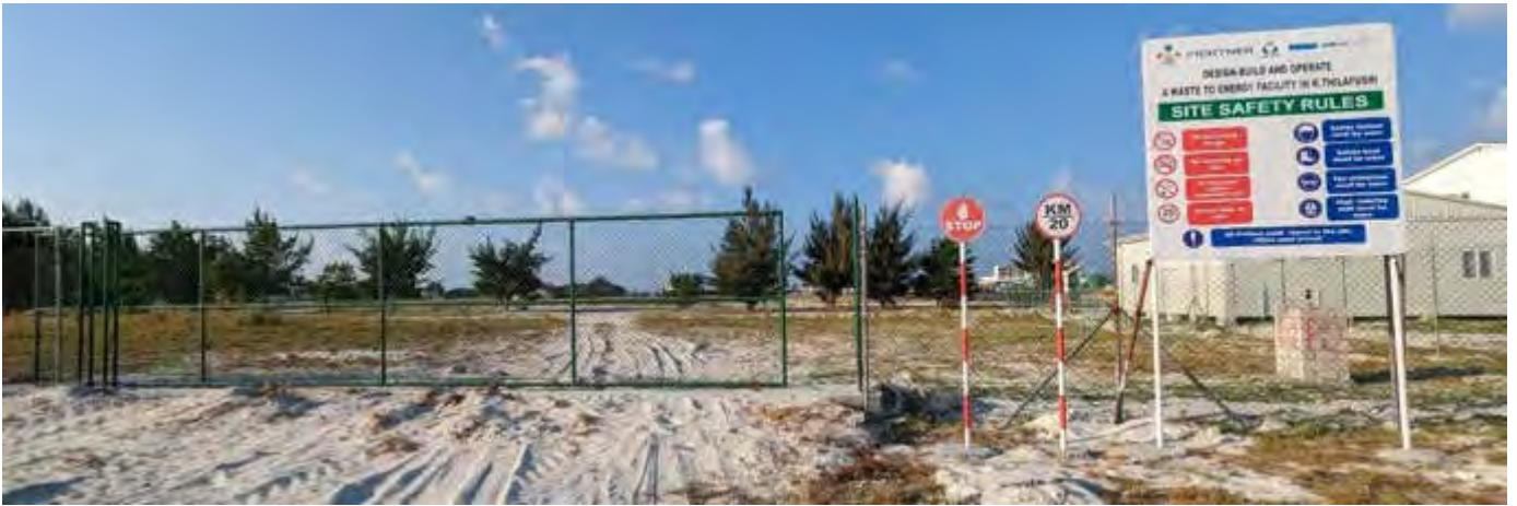
Photo 41 by Naif 27/02/23 17:18hrs Extra gate established for vehicles and materials movement.
