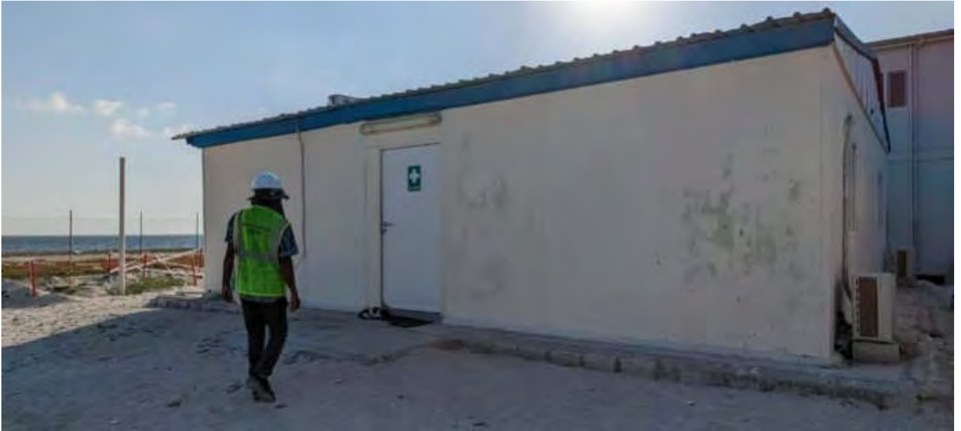
Photo 30 by Naif 27/02/23 16:40hrs. First aid room established, and doctor on site during working hours.
