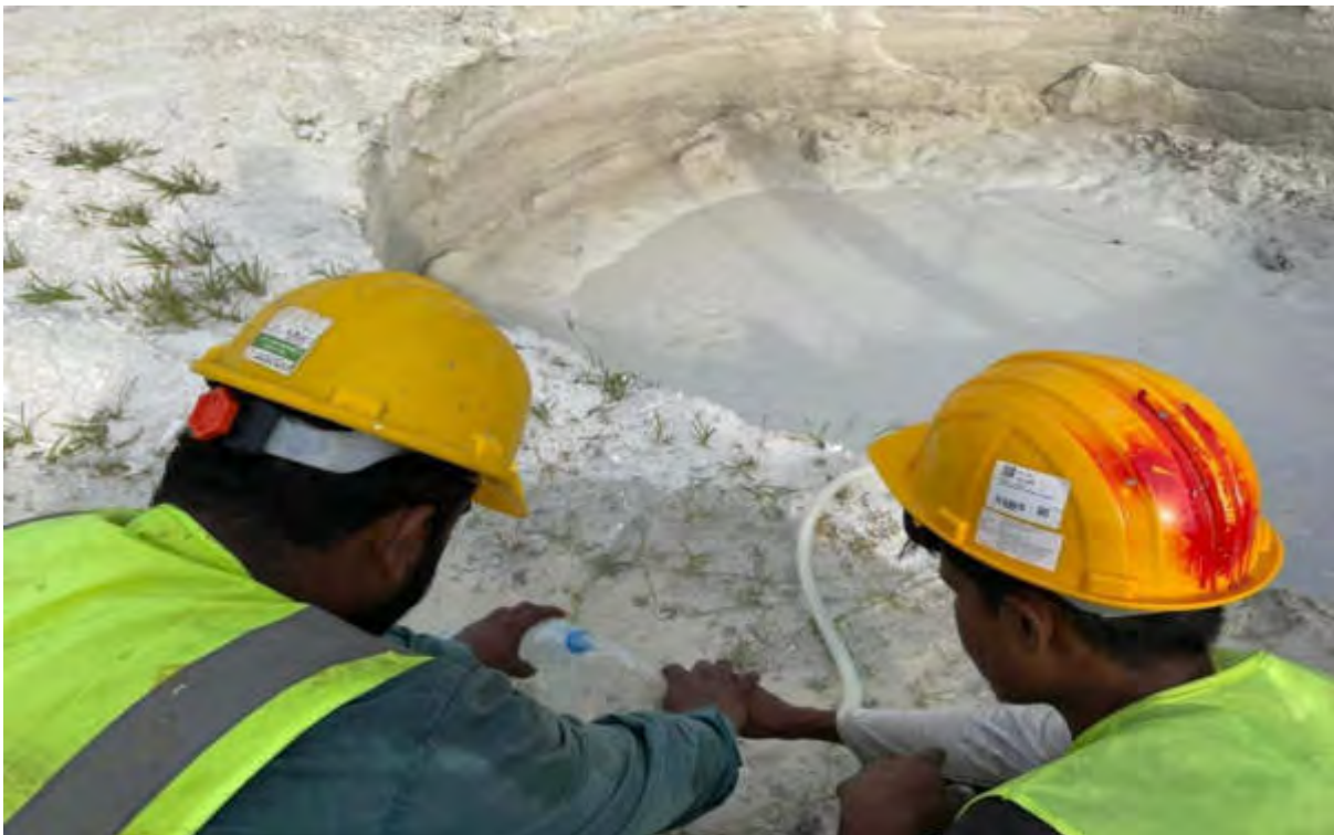
Ground water samples have been collected for dewatering permit.
