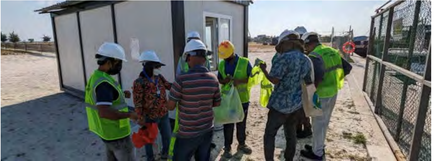
Photo 07 by Naif 27/02/23 15:47hrs. PPE issued to visitors prior to access to site.
