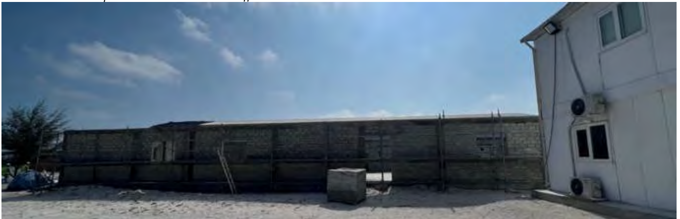
Photo 04 by Naahee 18/02/23 09:34hrs. Construction of mess hall ongoing.
