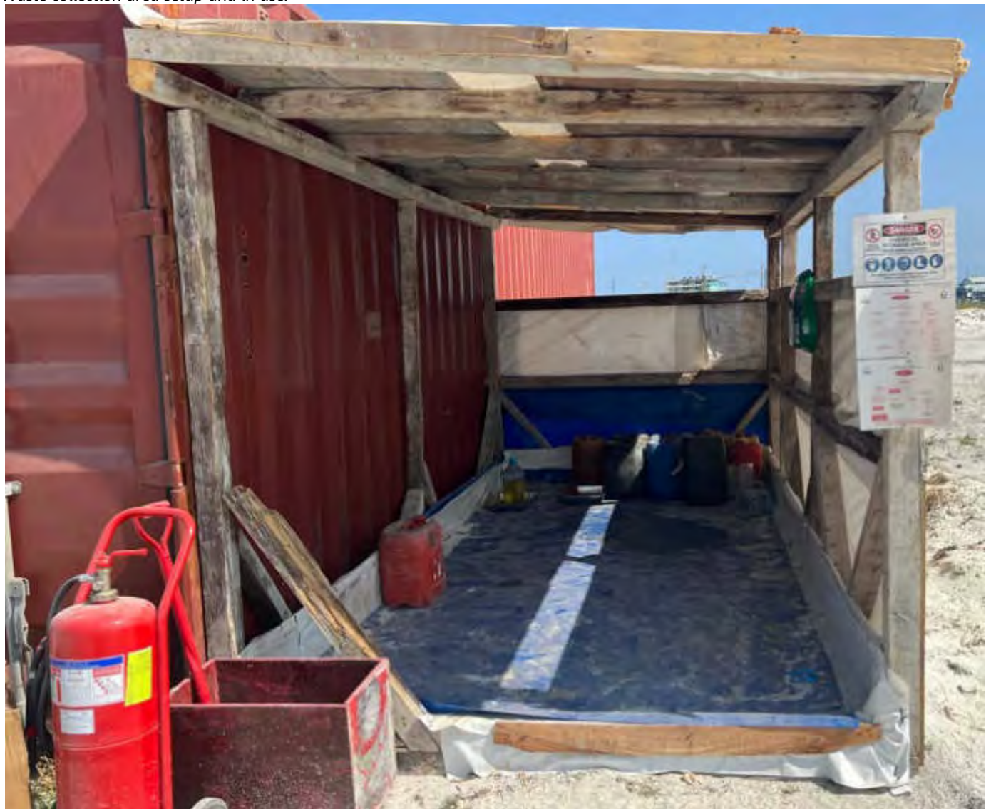
Photo 26 by Naahee 18/02/23 09:56hrs Hazardous chemical storage not completed yet, work is on going and to be completed soon.
