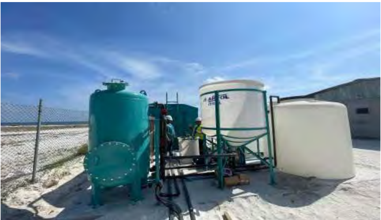
Installation of the WWTP was completed
