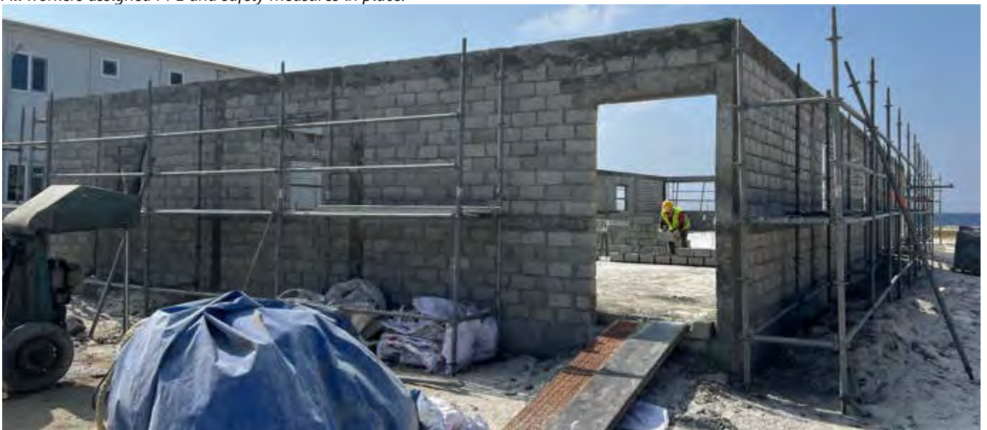
Photo 08 by Naahee 18/02/23 09:37hrs. Construction ongoing for workers mess hall.
