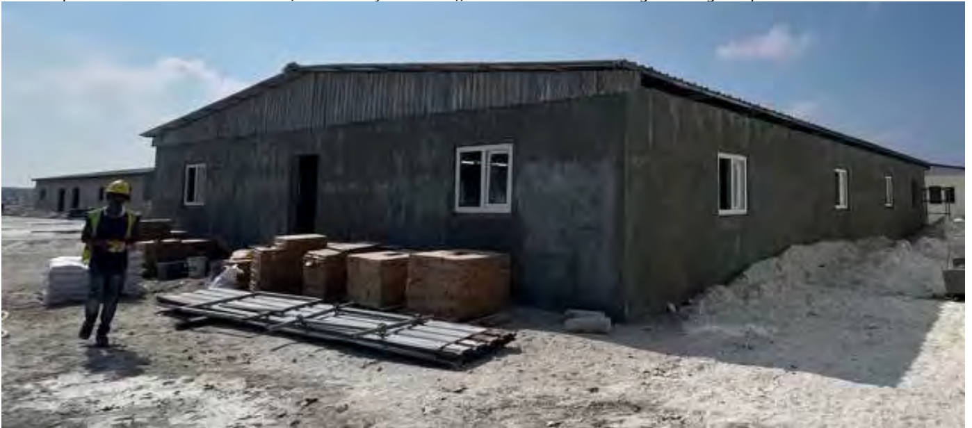
Photo 10 by Naahee 18/02/23 09:38hrs. Prayer hall and recreation center under construction.
