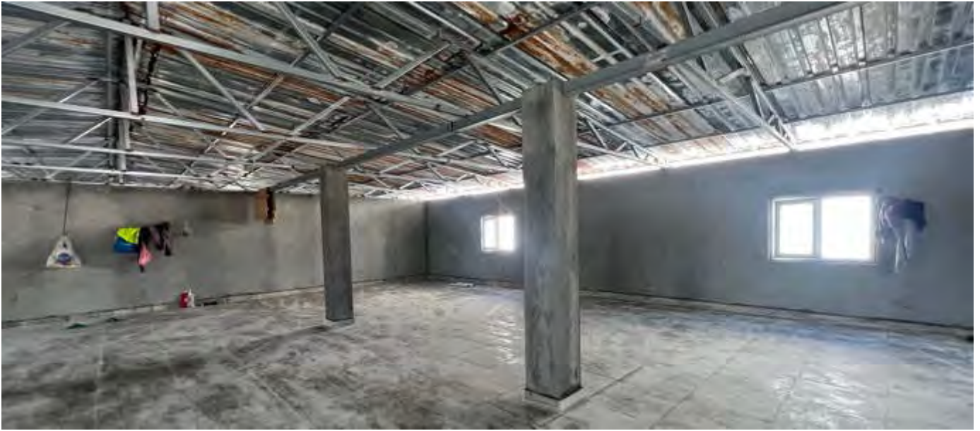
Photo 11 by Naahee 18/02/23 09:39hrs. Prayer hall under construction.
