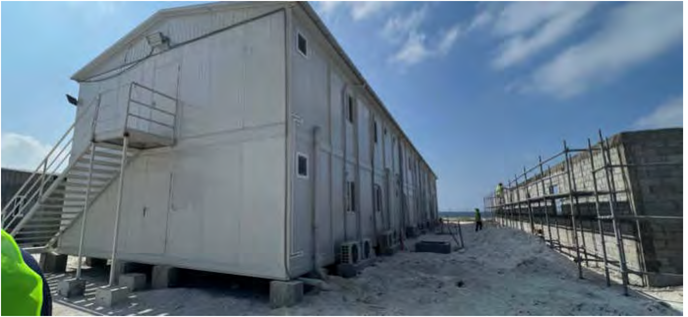
Photo 09 by Naahee 18/02/23 09:38hrs. Fire escape stairs located on both ends of the hallway in the staff accommodation building, building completed.
