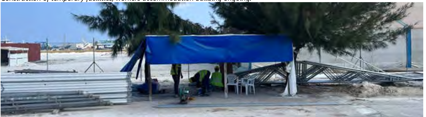
Photo 13 by Naahee 18/02/23 09:40hrs. Metal fabrication work ongoing, all workers with PPE.
