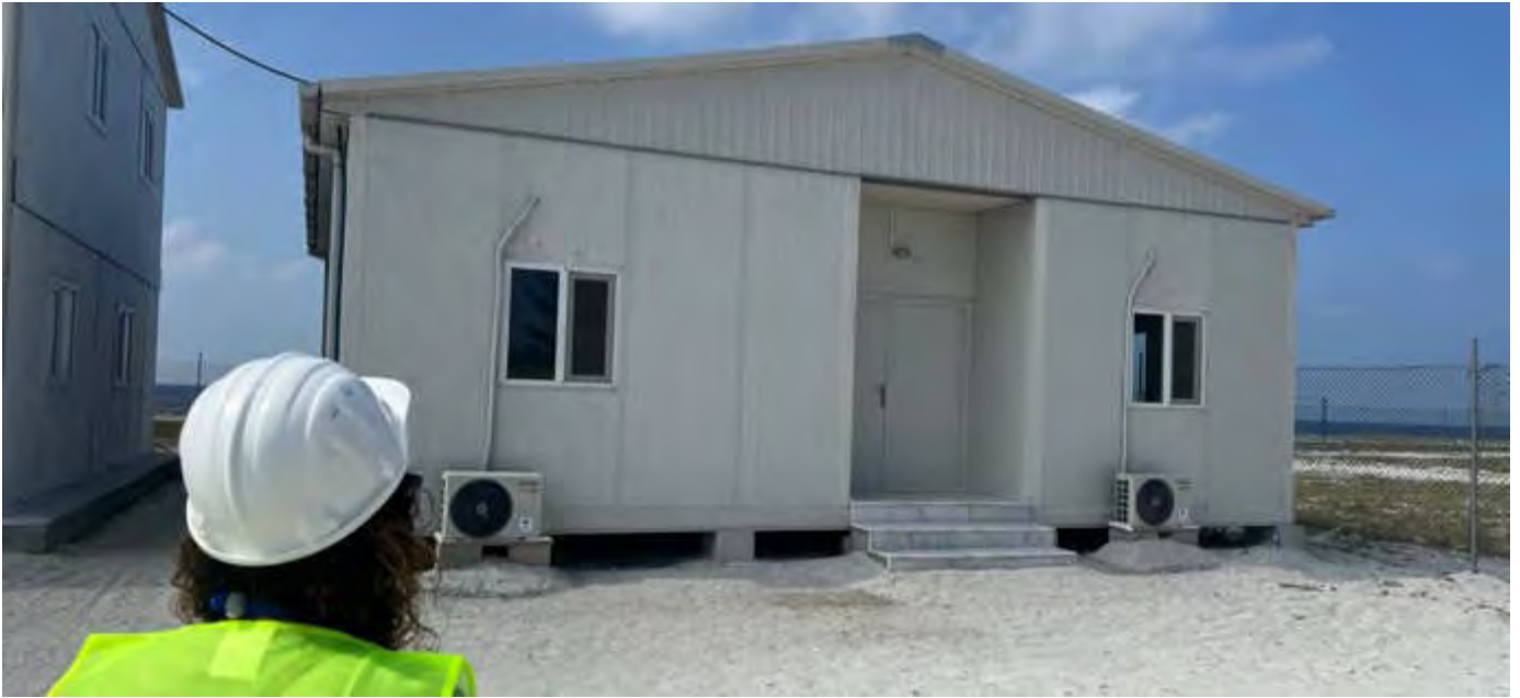
Photo 01 by Naahee 18/02/23 09:33hrs. E.R. office and accomidation building completed.
