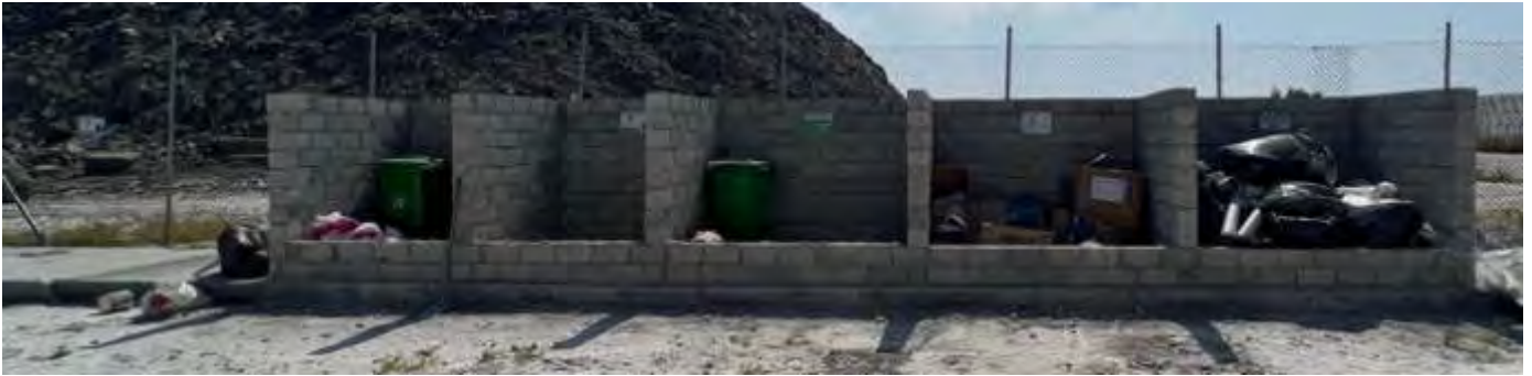
Photo 25 by Naahee 18/02/23 09:58hrs Waste collection area setup and in use.
