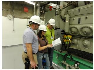
frequency depends on the manufacturer, how often the generator is used and your work environment. Typically, it is recommended you change the oil after 100 hours of operation, especially if the generator uses diesel.
