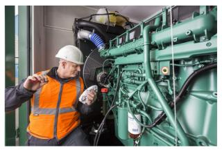
The oil and filter must also be changed at acclaimed time intervals. Check with the engine manufacturer for procedures for draining the oil and replacing the oil filter and their disposal is to be done appropriately to avoid environmental damage or liability.
