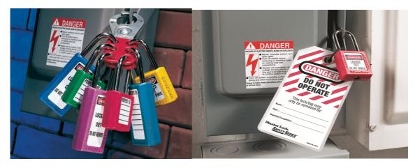
Test that the isolation is effective by 'trying' to reactivate the plant without exposing the tester or others to risk. Failure to reactivate the plant means that the isolation procedure is effective and that all stored energies have dissipated.
