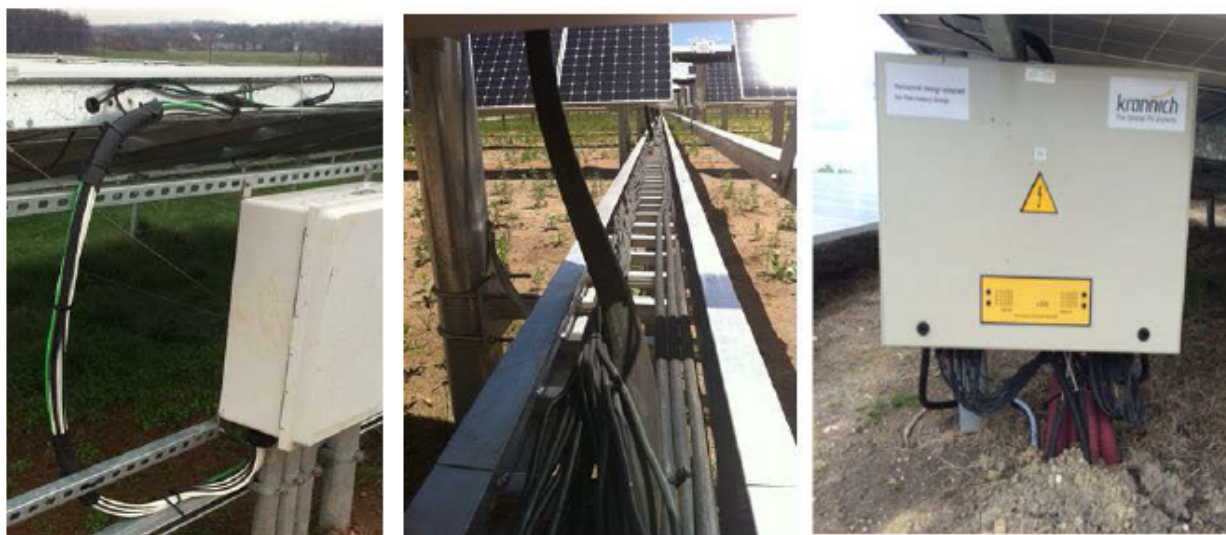
Maintenance of wire management systems depend on plastic wire ties and grommets, which can break or pinch wires (left); exposure to sunlight; wind and weight of ice (center); and access by chewing rodents (right).
