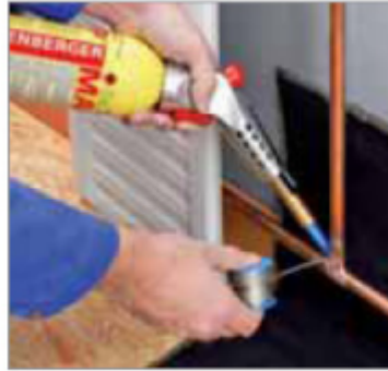
Soft Soldering central heating pipe Flame beating action on joint
