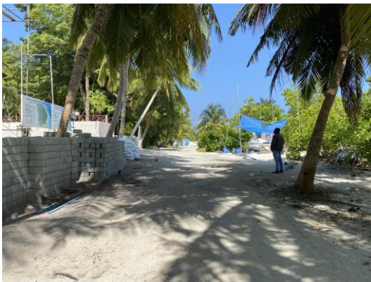
Figure 14: Access road condition
