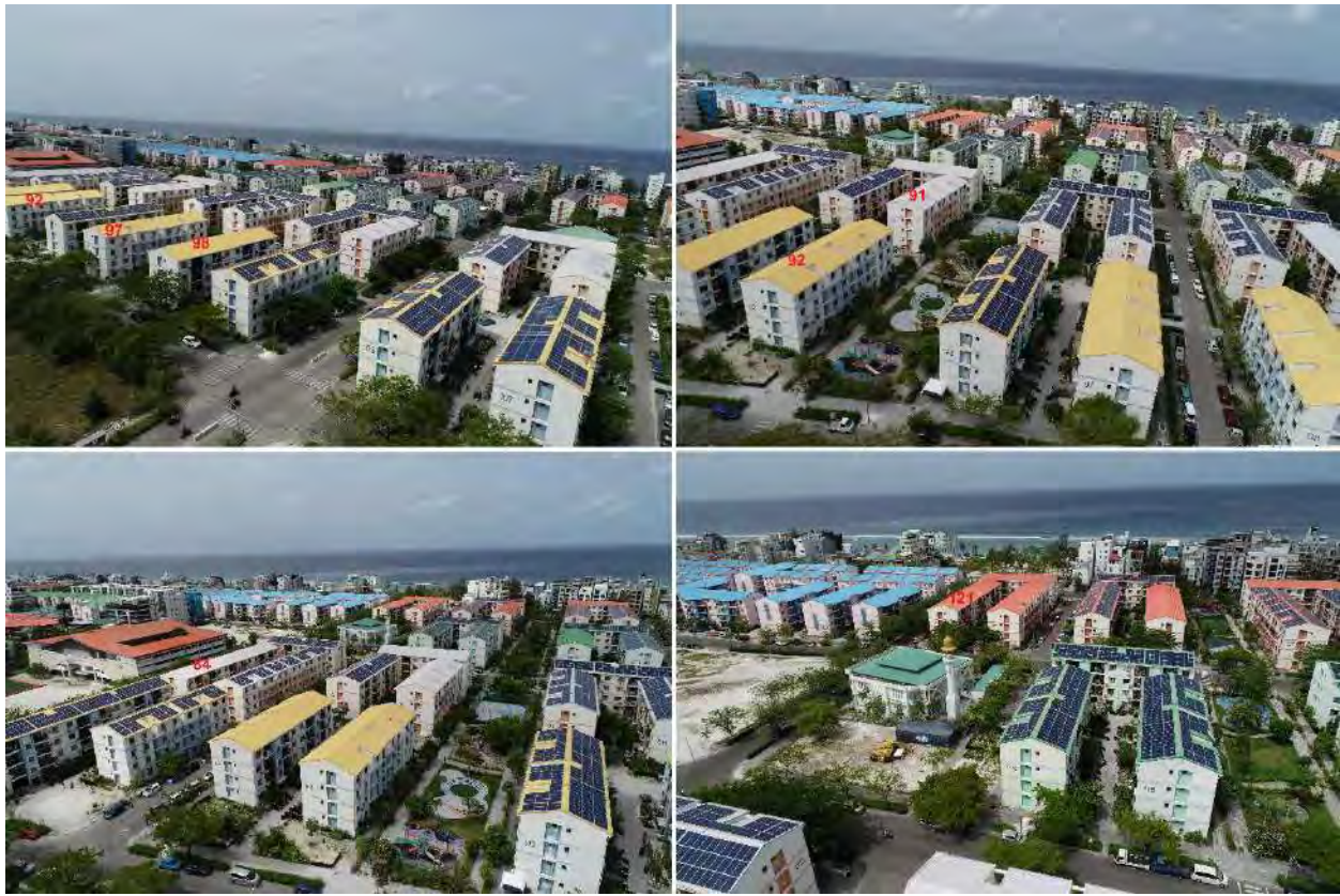
Figure 6-5: Rooftop installation area
