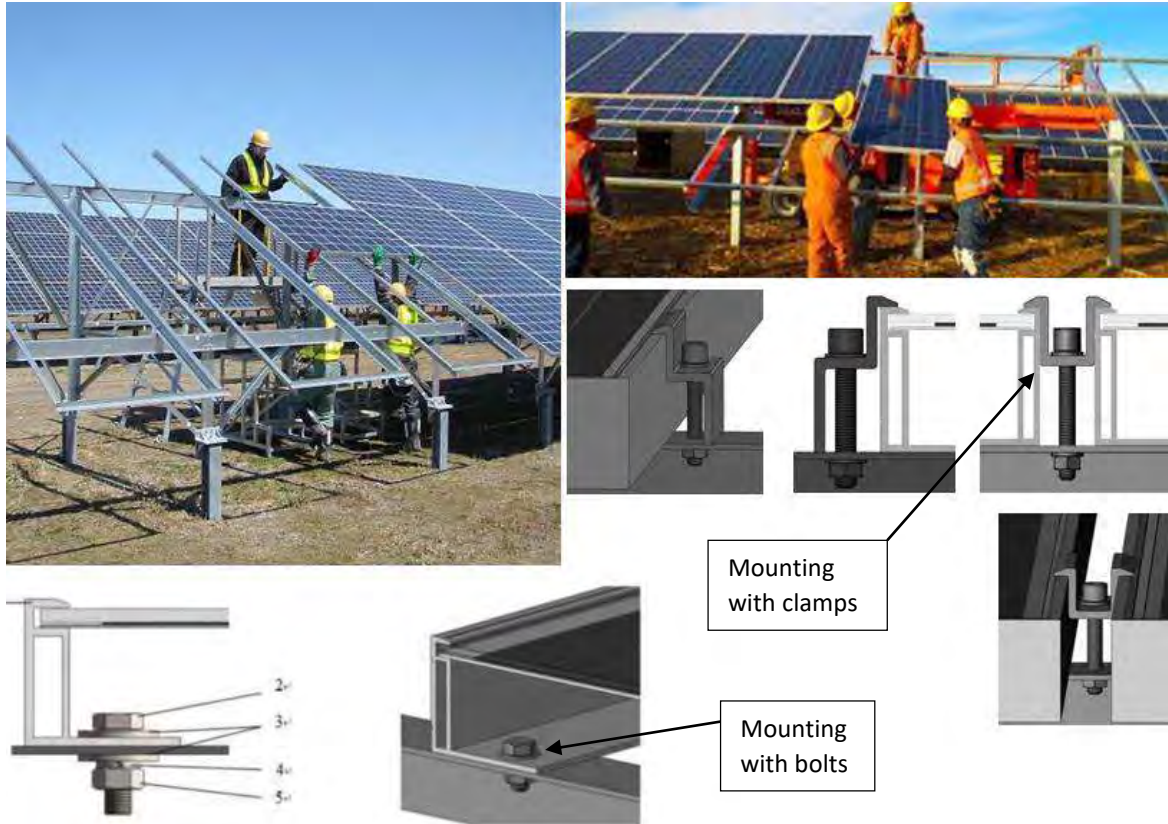
Figure 3-17: Installation of PV modules
