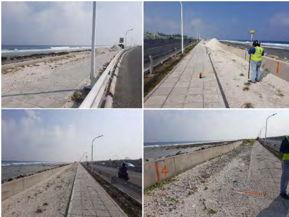
Figure 6-2: Eastern side of the link road
