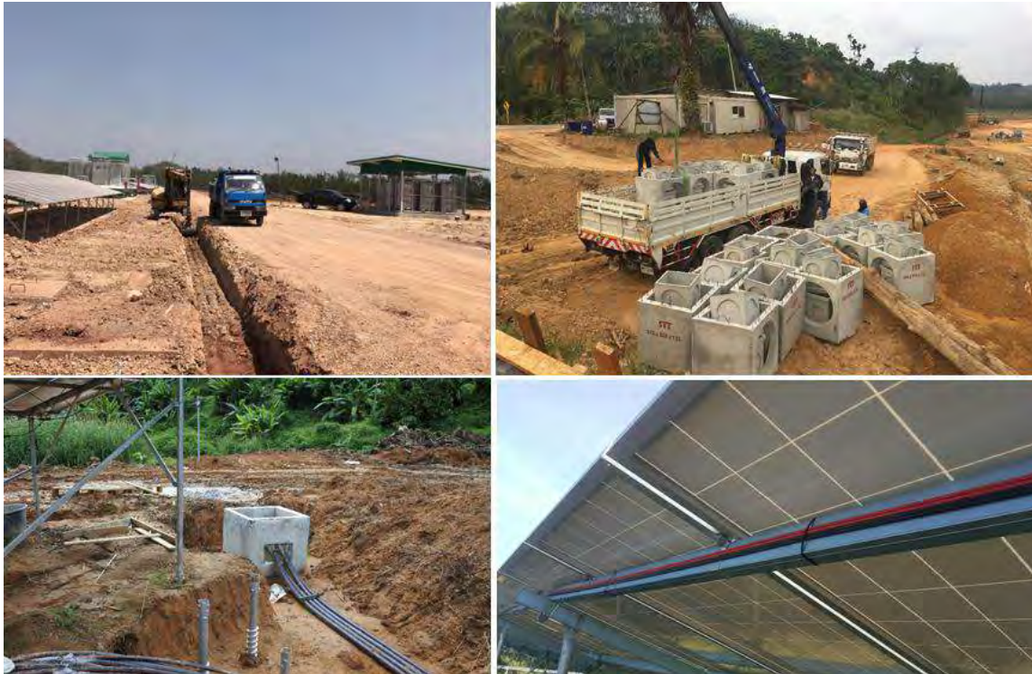
Figure 3-15: Cable connection and installation (reference pictures of similar works)
