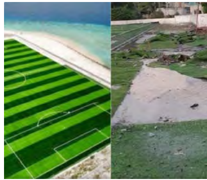
Figure 65: Soccer ground of Lh.Kurendhoo was damaged due to wave surge on 24 th Sept 2021.
