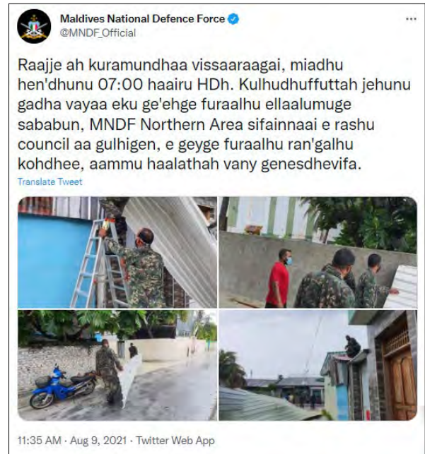
Figure 52: MNDF reported response to damages due to strong gust winds during the morning of 9 th August at Hdh Kulhudhufushi
