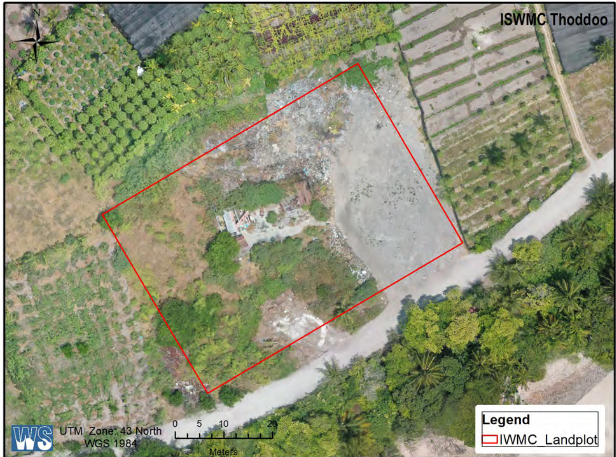
Figure 13: Photos of Thoddoo IWMC site
