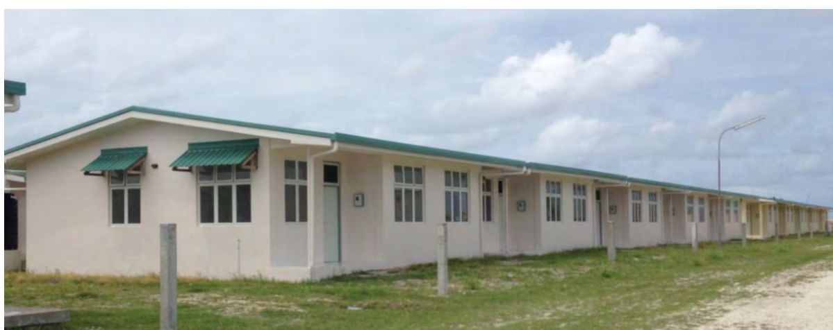
FIGURE 2 SINGLE STORY HOUSES, PROVINCE HOUSING DEVELOPMENT PROJECT
