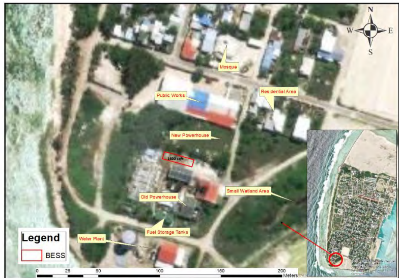
FIGURE 3 THINADHOO BESS LOCATION
