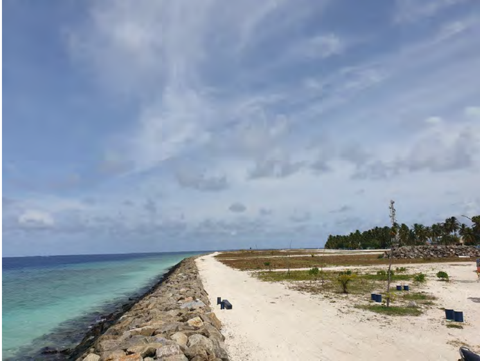
Figure 3 Photo of the installation site
