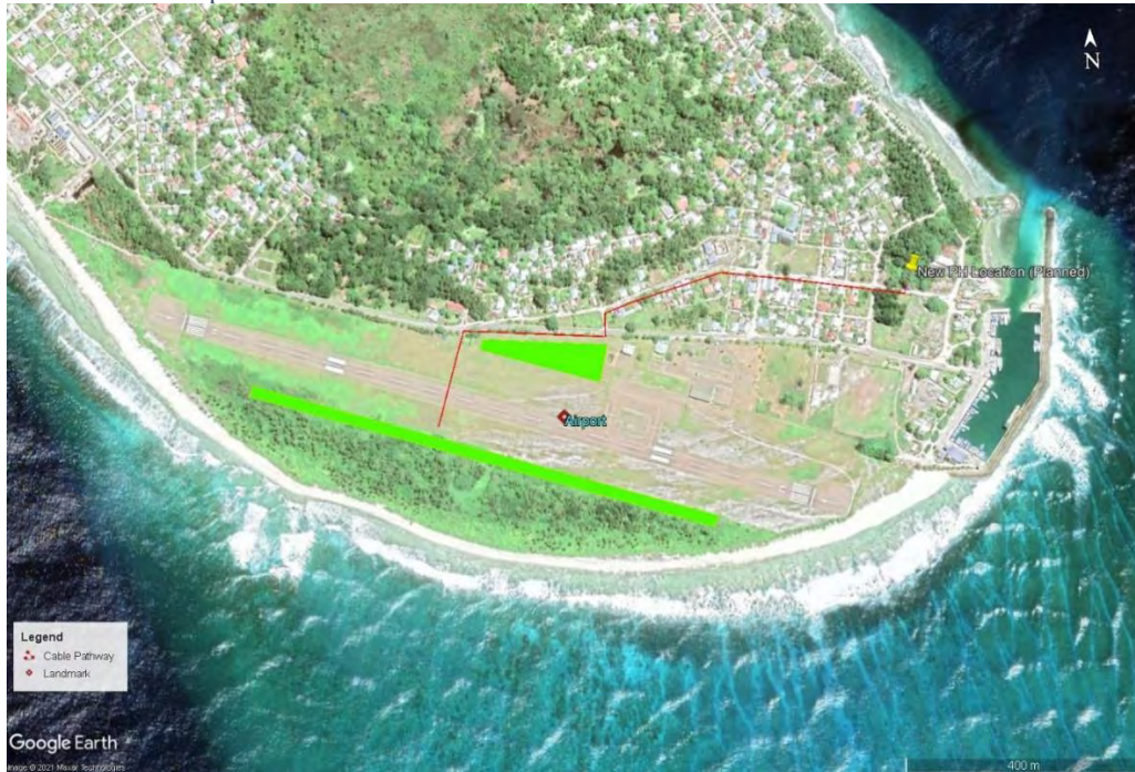
FIGURE 7 LANDMARKS NEAR GRID UPGRADING PATHWAY FUVAHMULAH
