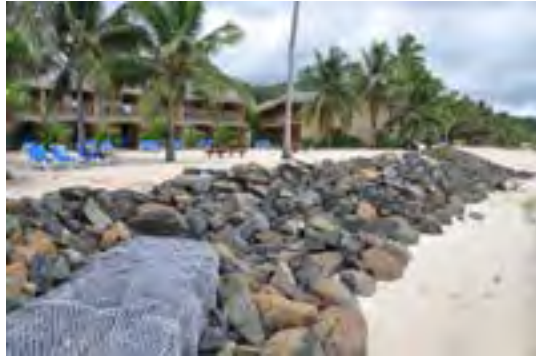
Revetment (sloping) seawall
