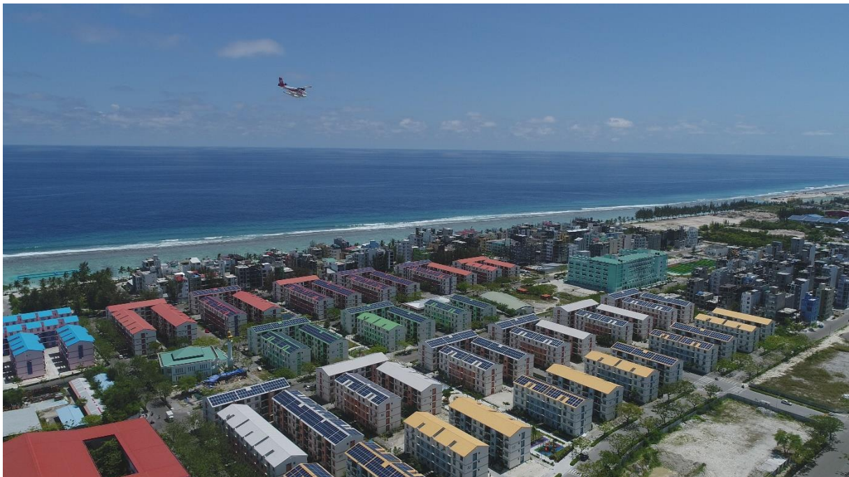
Figure 1 Solar Pv installed at selected blocks of 1000 housing units
