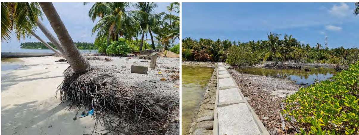
Figure 17. South eastern corner area
