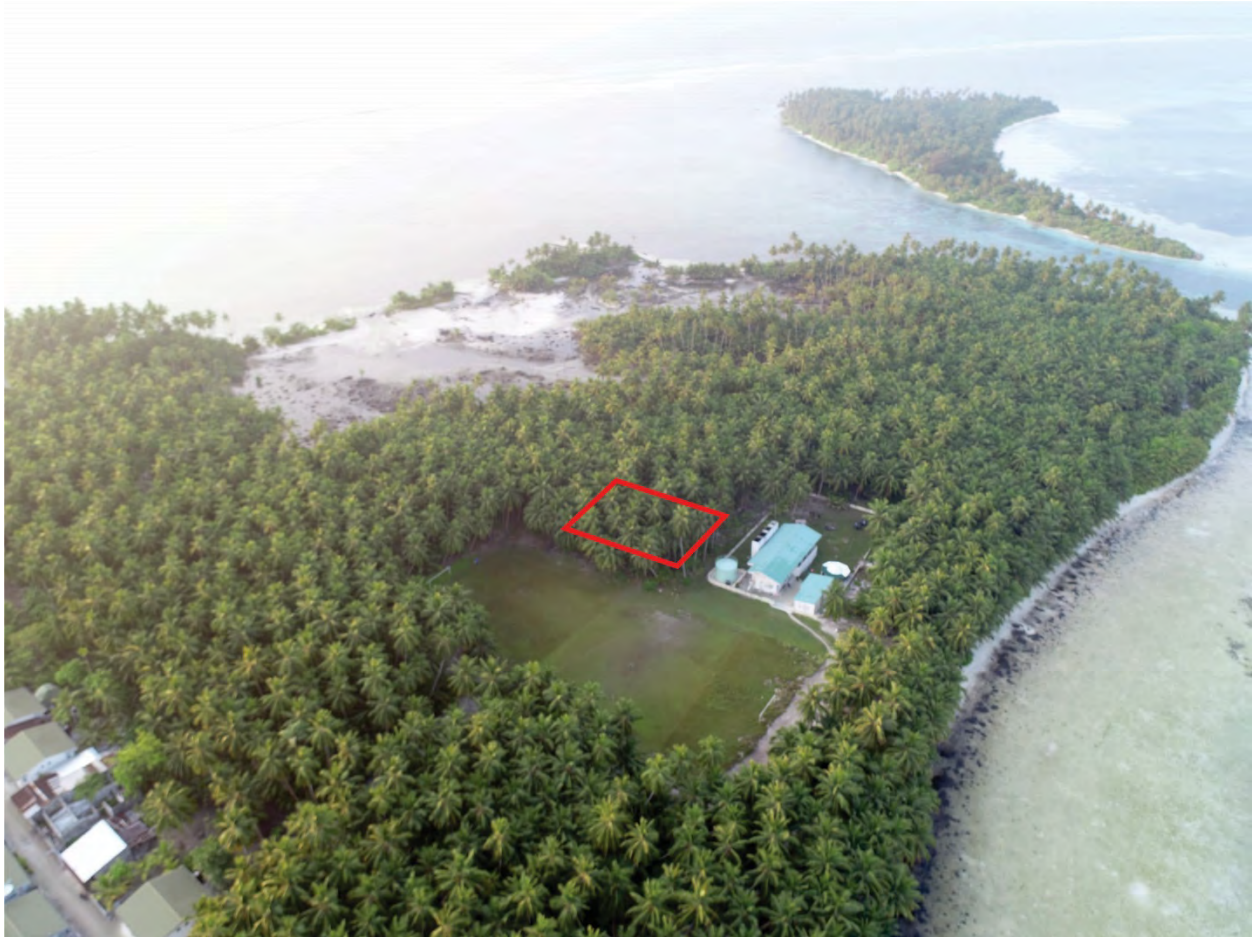
Figure 20. Drone image showing proximity of IWRMC site to encroaching marsh land
