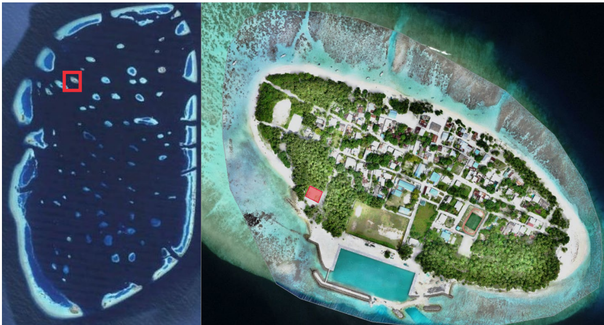
Figure 1. Location of Rinbudhoo in Dhaalu Atoll (left, red highlight) and existing IWRMC and project site (right, red highlight)
