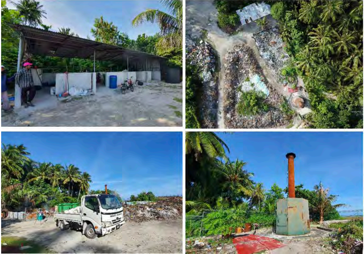
Figure 8 Waste separation bays, collection trucks and incinerator (burner).
