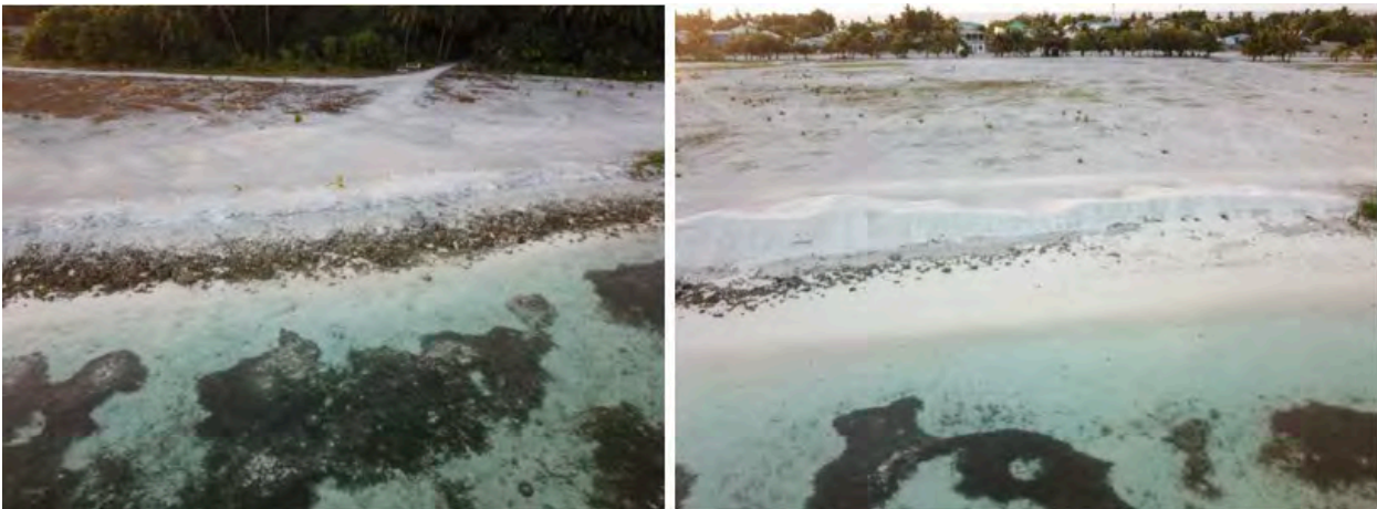
Figure 13 Sediment being eroded as there was no protection put in place.
