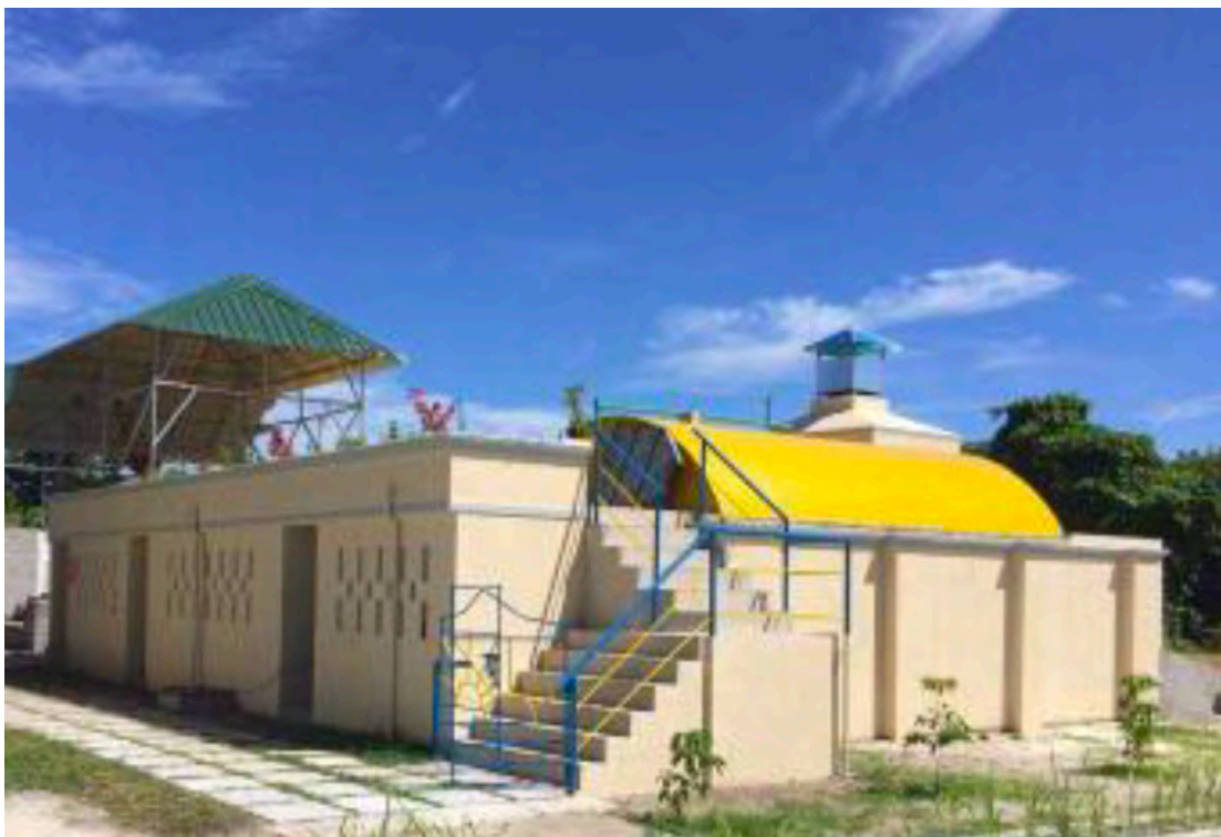
Figure 7 Example of AD plant installed in a resort hotel, Reethifaru, Baa atoll (source: BIOGEN, India)
