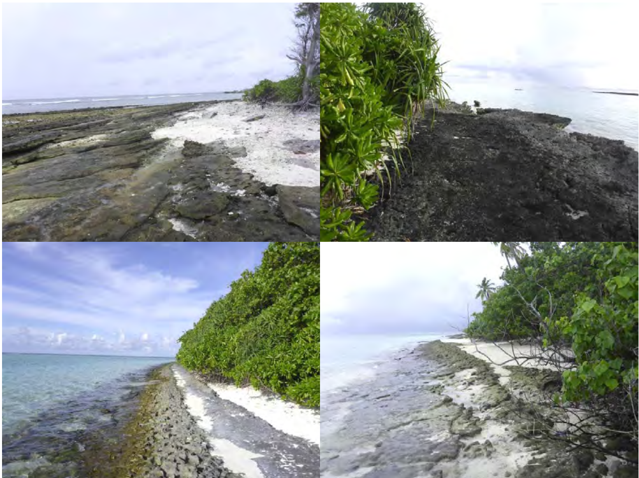
Figure 3.14 Beach rock as a natural revetment in strong wave conditions: (a) Maalhos; (b) Mathiveri (c)Thoddoo and (d) Himandhoo
