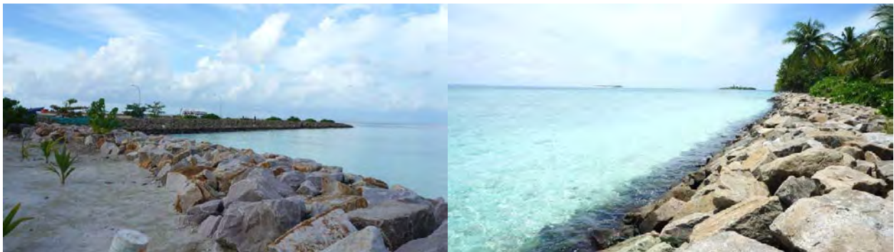
Figure 4.11 Revetment – Armor rock structures in Mathiveri and Rasdhoo
