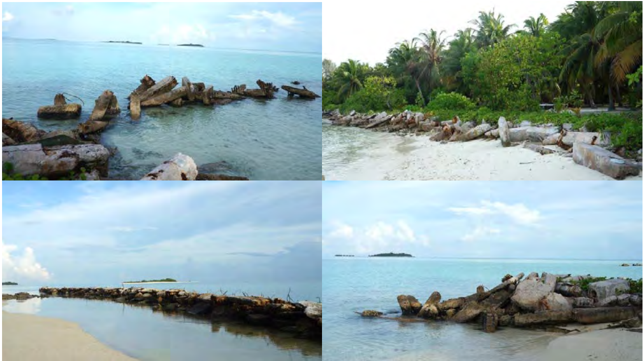
Figure 4.14: Ad hoc dumping of construction waste to mitigate erosion in Mathiveri Island. A range of measures including groynes, revetments and nearshore breakwater have been constructed using harbour demolition waste.
