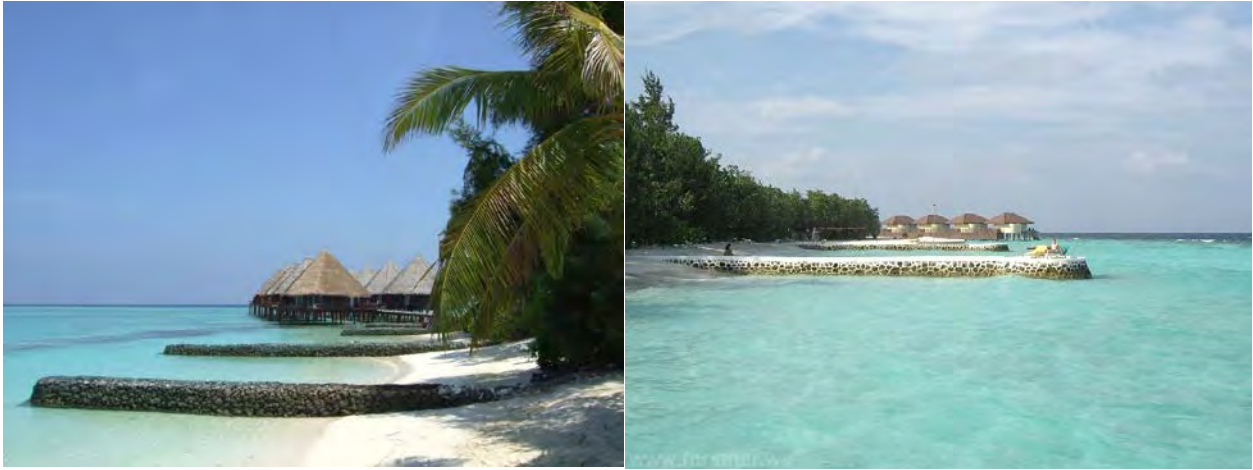
Figure 4.12 Groynes used for erosion mitigation in Velidhoo and Mayyafushi
