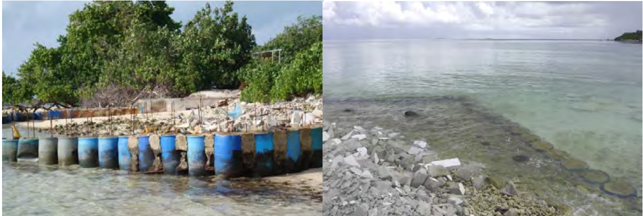
Figure 4.4 Example of improvised Seawall structures: concrete filled barrels in AA Bodufolhudhoo
