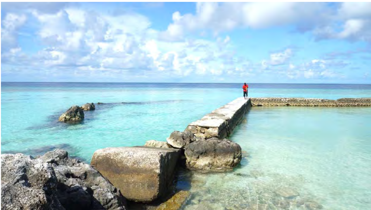
Figure 4.9 Break water design used prior to 2010s – sand cement bags from Thoddoo Island
