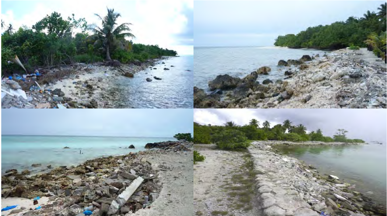
Figure 4.15 Construction waste used for erosion mitigation in (a, b) Thoddoo, (c) Ukulhas and (d) Bodufolhudhoo
