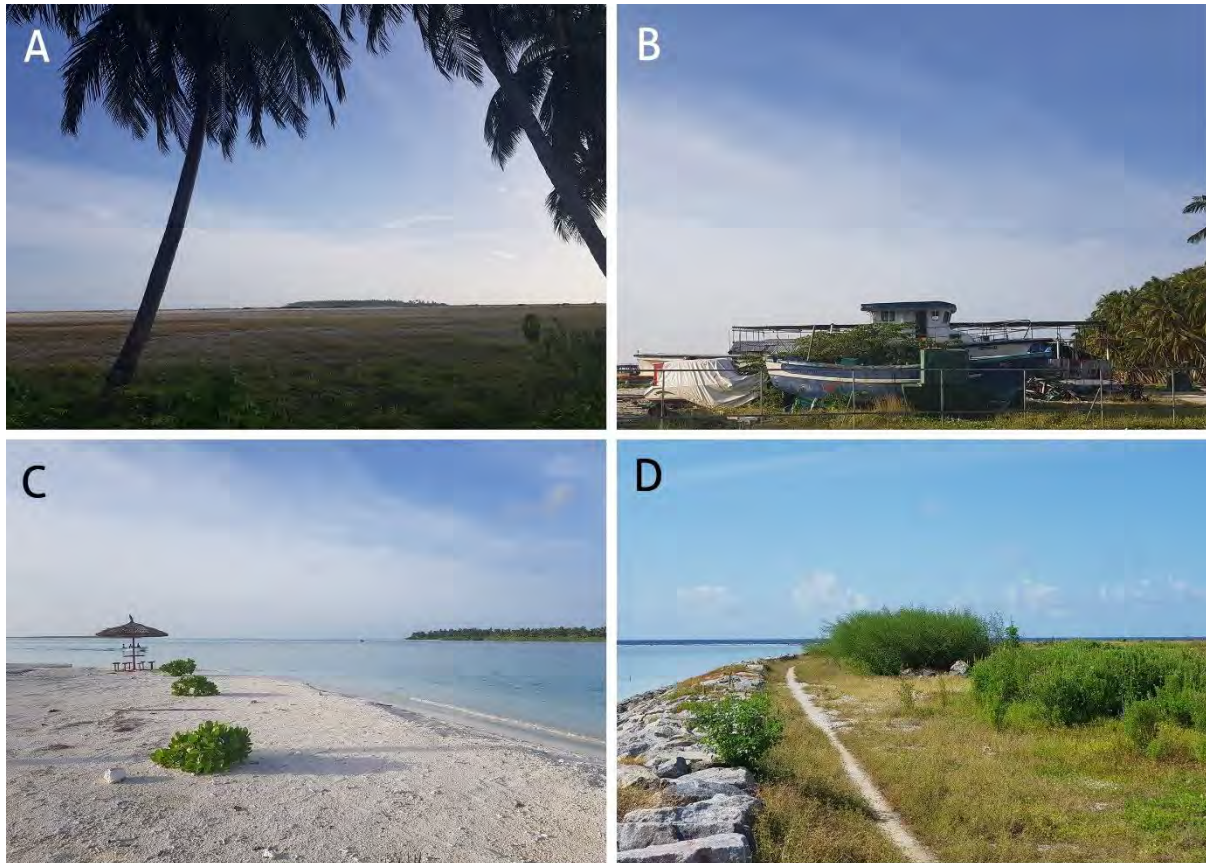
Figure 6 (A) Newly reclaimed area and coconut palms of the islands natural vegetation line (B) Boat building work (C) Area being developed as an artificial beach (D) Coastal protection of newly reclaimed area
