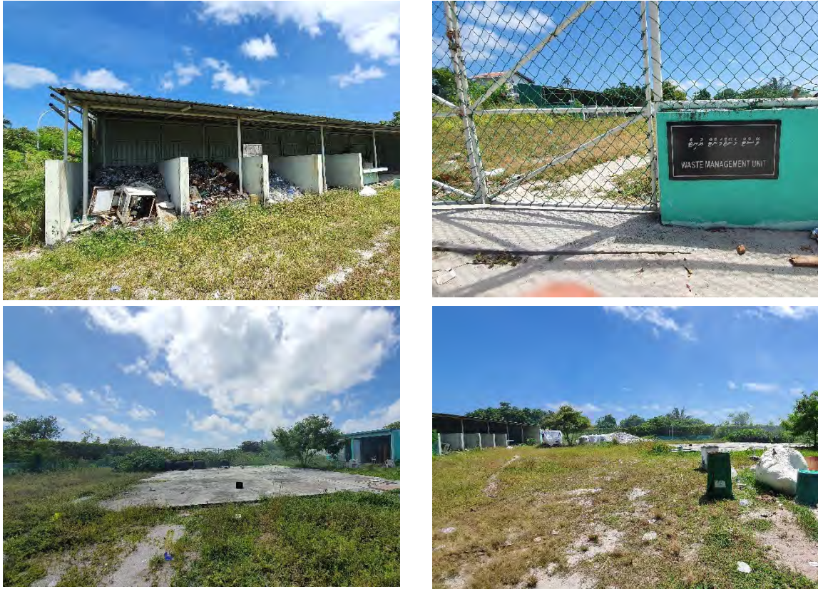
Figure 6. Waste site enclosed by fence and site is closed. Waste is currently dumped outside the site
